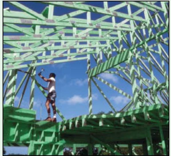
*FrameGuard® treatment keeps lumber looking cleaner and brighter during storage, construction, and beyond. This is especially important to truss and component manufacturers whose end products tend to be exposed to the elements longer than other framing materials.*
